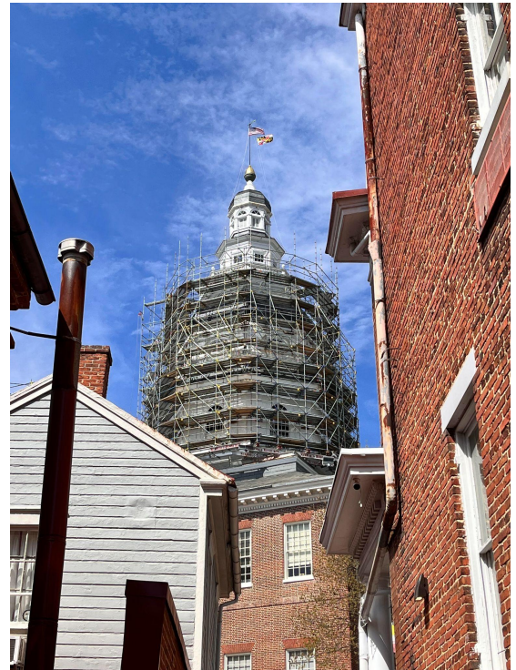
Scaffolding erected around State House dome, in progress May 2022.
